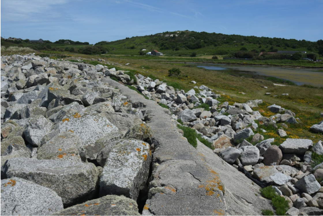
Figure 9.14: Showing the crest and crown wall of the Great Popplestone rock revetment (Great Pool can be seen to the right hand side)
