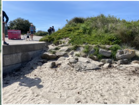
H SITE 8. Quay eroded section
