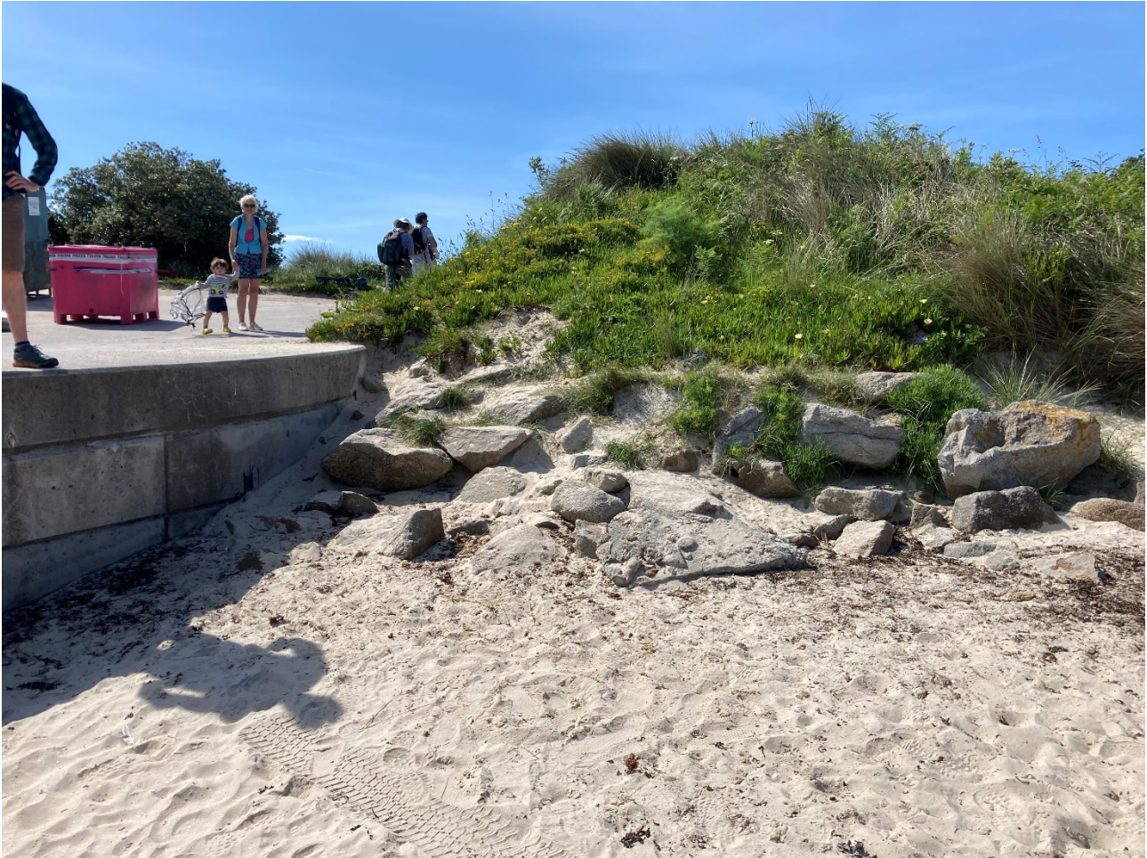
Figure 9.20: Showing erosion of the embankment adjacent to the Green Bay quay
