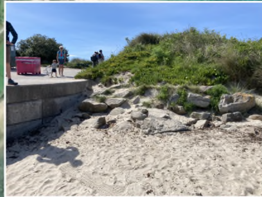
H SITE 8. Quay eroded section
